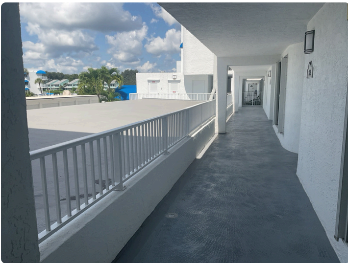
Typical walkway railing
