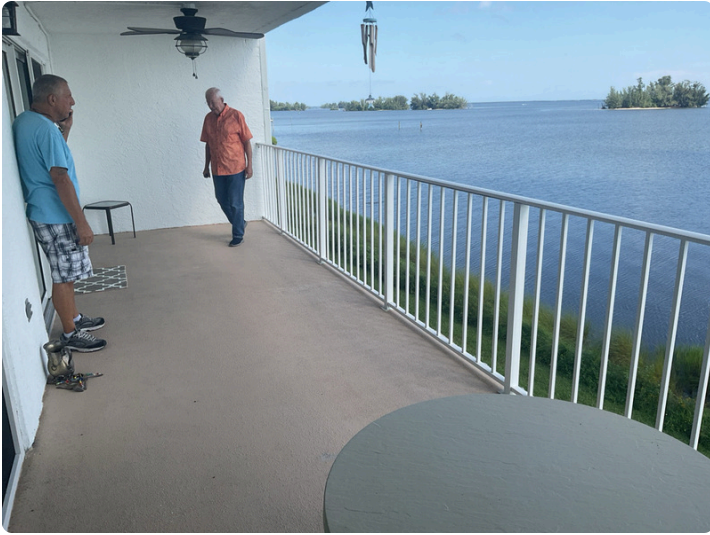
Typical balcony railing
