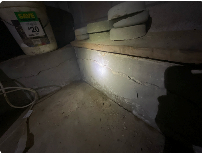
Spalled/cracking concrete
