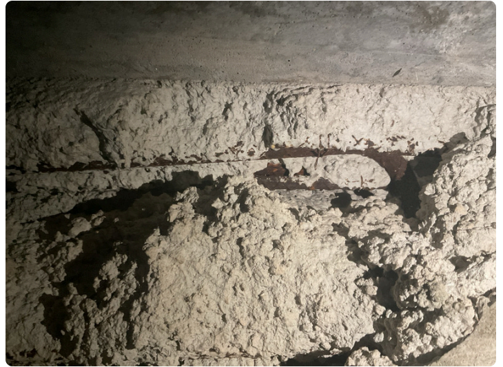
Exposed rebar
