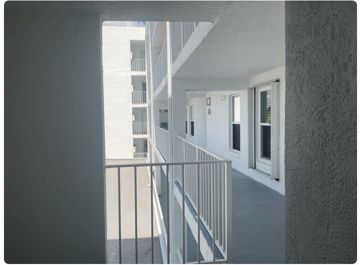
Typical walkway railing
